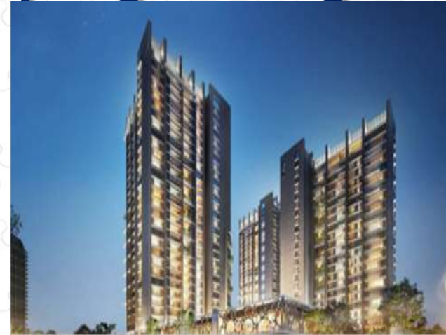
PONDOK INDAH RESIDENCE - JAKARTA
