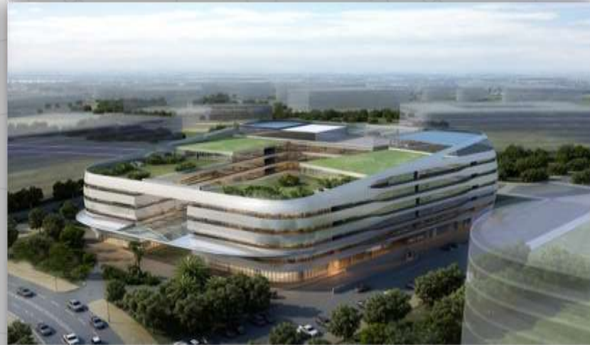
GREEN OFFICE PARK 3-TANGERANG
