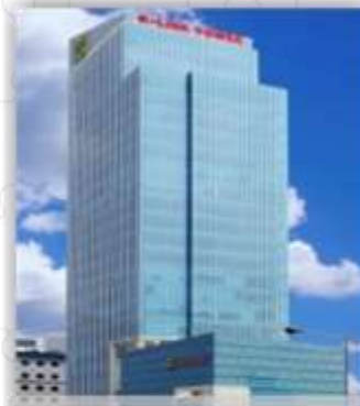
K-LINK TOWER JAKARTA
