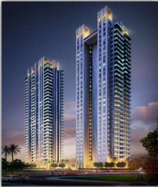
VERDE II CONDOMINIUMS JAKARTA
