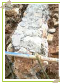
Perapian dinding penahan tanah Tidying up of the retaining wall
