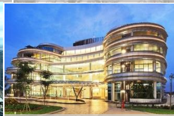
GREEN OFFICE PARK 1 - TANGERANG
