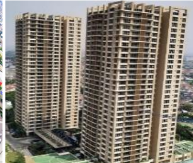
PONDOK INDAH RESIDENCE - JAKARTA
