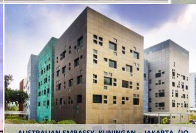
AUSTRALIAN EMBASSY, KUNINGAN - JAKARTA. (JO PROJECT)
