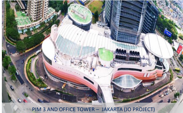
PIM 3 AND OFFICE TOWER - JAKARTA (JO PROJECT)
