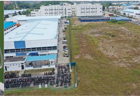
SIMATELEX PHASE 4 - BATAM
