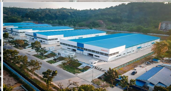
SIMATELEX PHASE 3 - BATAM
