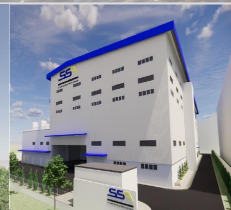
SSA PLANT - CIKARANG
