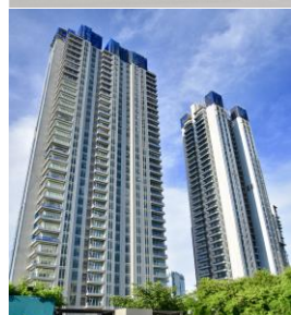
VERDE II CONDOMINIUMS JAKARTA
