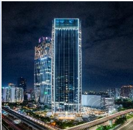
DASWIN OFFICE TOWER - JAKARTA. (JO PROJECT)
