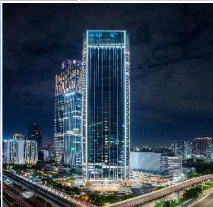
DASWIN OFFICE TOWER - JAKARTA. (JO PROJECT)
