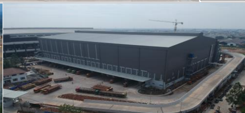
MMP13 WAREHOUSE – PD UNGU
