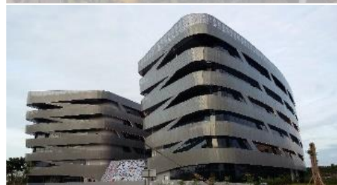
GREEN OFFICE PARK 9 BSD - TANGERANG
