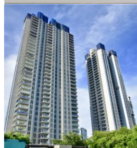
VERDE II CONDOMINIUMS JAKARTA
