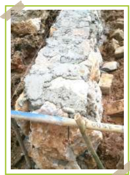
Perapian dinding penahan tanah Tidying up of the retaining wall
