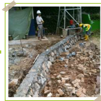
Pemasangan bobokan bored pile Installation of bored pile rubble
