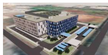
■ BNDC - BCA Data Center
