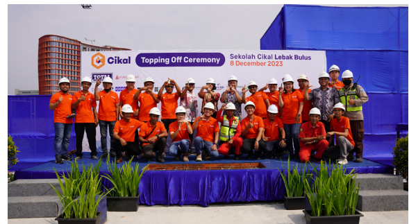
PROSESI PENUTUPAN ATAP (TOPPING OFF) PROYEK SEKOLAH CIKAL LEBAK BULUS TAHAP 2 A TOPPING OFF CEREMONY AT SEKOLAH CIKAL LEBAK BULUS 2ND PHASE PROJECT
