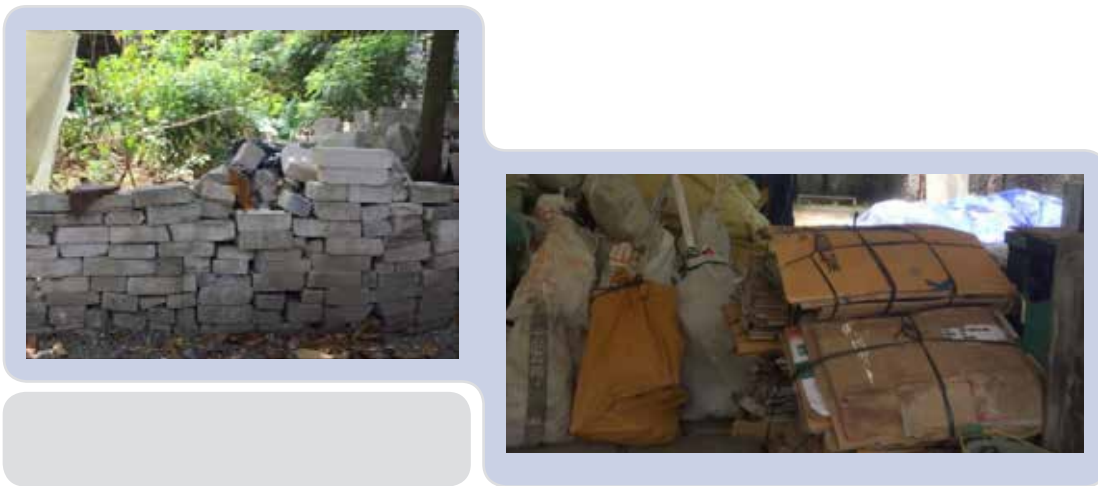
Pemanfaatan dan Pengelolaan Sampah Konstruksi Proyek Sequis Towe di Lokasi Penampungan Sampah di Luar Area Proyek / Waste Utilization and Management of Sequis Tower Project Construction at Waste Collection Sites Outside the Project Area
